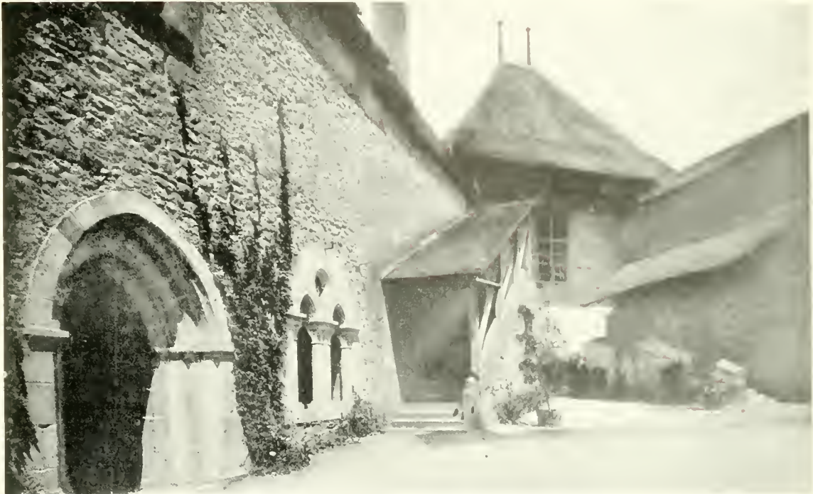
CHILLON—COURT AND STAIRS OF HONOR
